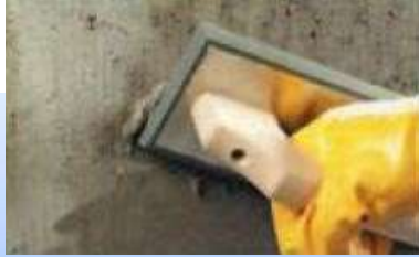
Finishing Porous Concrete in Precast Concrete
